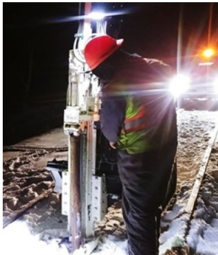
Drilling with Geoprobe Rig
